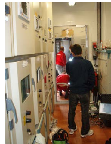
Inside the container during installation
