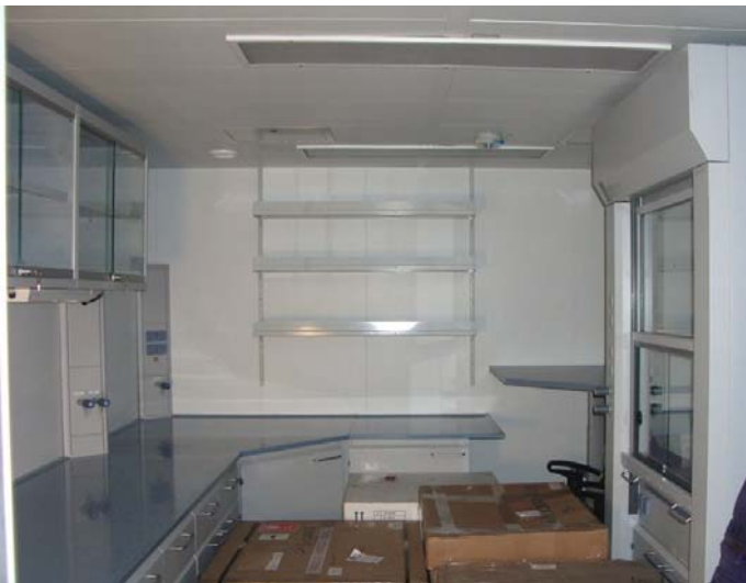
Internal outfitting of the Laboratory module
